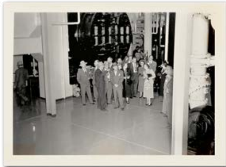
About 150 people toured the Osage Power Plant during its open house on May 12, 1950. With construction delayed by the war, the plant represented the first major expansion of the company’s power generation facilities.
