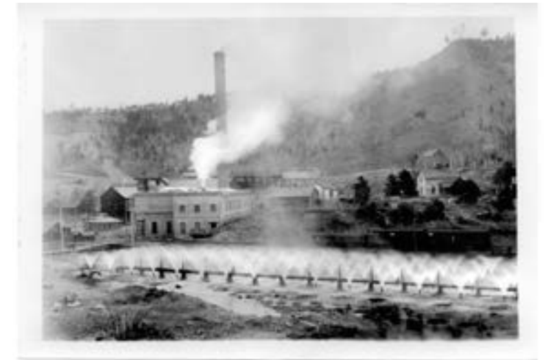
Before cooling towers had been developed at the Pluma Plant, the hot water from the steam vented through the generators was sprayed over a pond beside Whitewood Creek.
