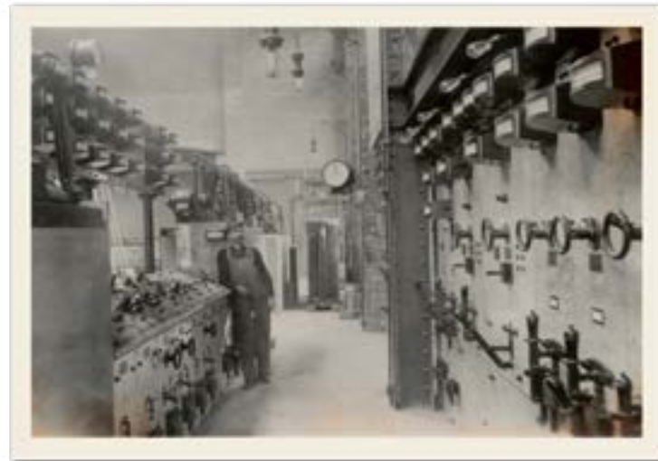
In the central room of the Pluma Plant in 1910, employees monitored the temperatures and pressures inside the boilers and steam turbine generators.
