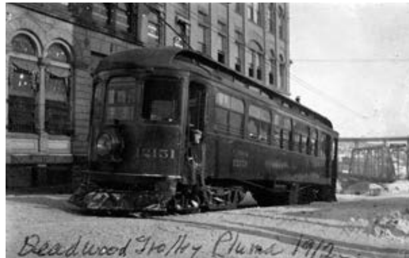
In 1901 electric cars replaced a steam locomotive on the light rail that ran between Lead and Deadwood. The Belt Light and Power Company of Lead converted 11,000 volts AC to 600 volts DC to power the Burlington inter-urban trolleys. The company produced the power at the Pluma plant.
