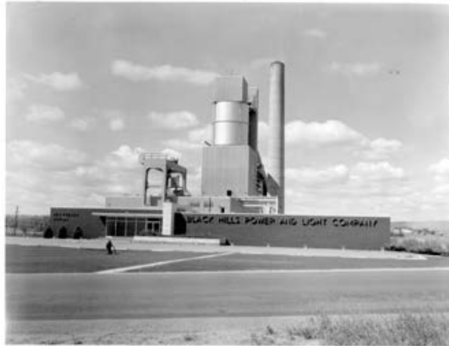
Ben French Power Plant began commercial operations in January 1961. Early on, the Ben French Power Plant primarily provided system stabilization rather than base load power.
