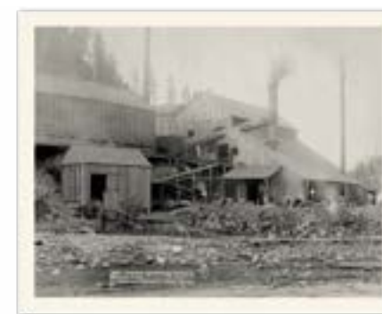
The pan and shovel days of the gold rush were gone by the late 1880s. The Deadwood and Delaware Smelter was the largest reduction plant in the world when it opened. Gold and silver worth nearly $2 million a year (approximately $52.2 million in 2018 dollars) were melted from massive quantities of ore excavated by hard rock miners.
