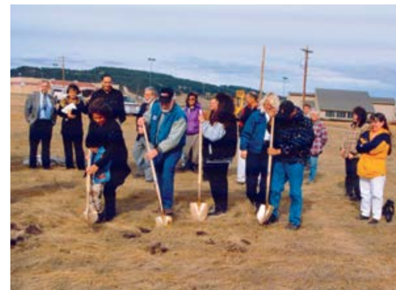
Community leaders joined company employees for Black Hills FiberCom's groundbreaking. Fast-tracking construction, the company began offering service in the fall of 1999.
