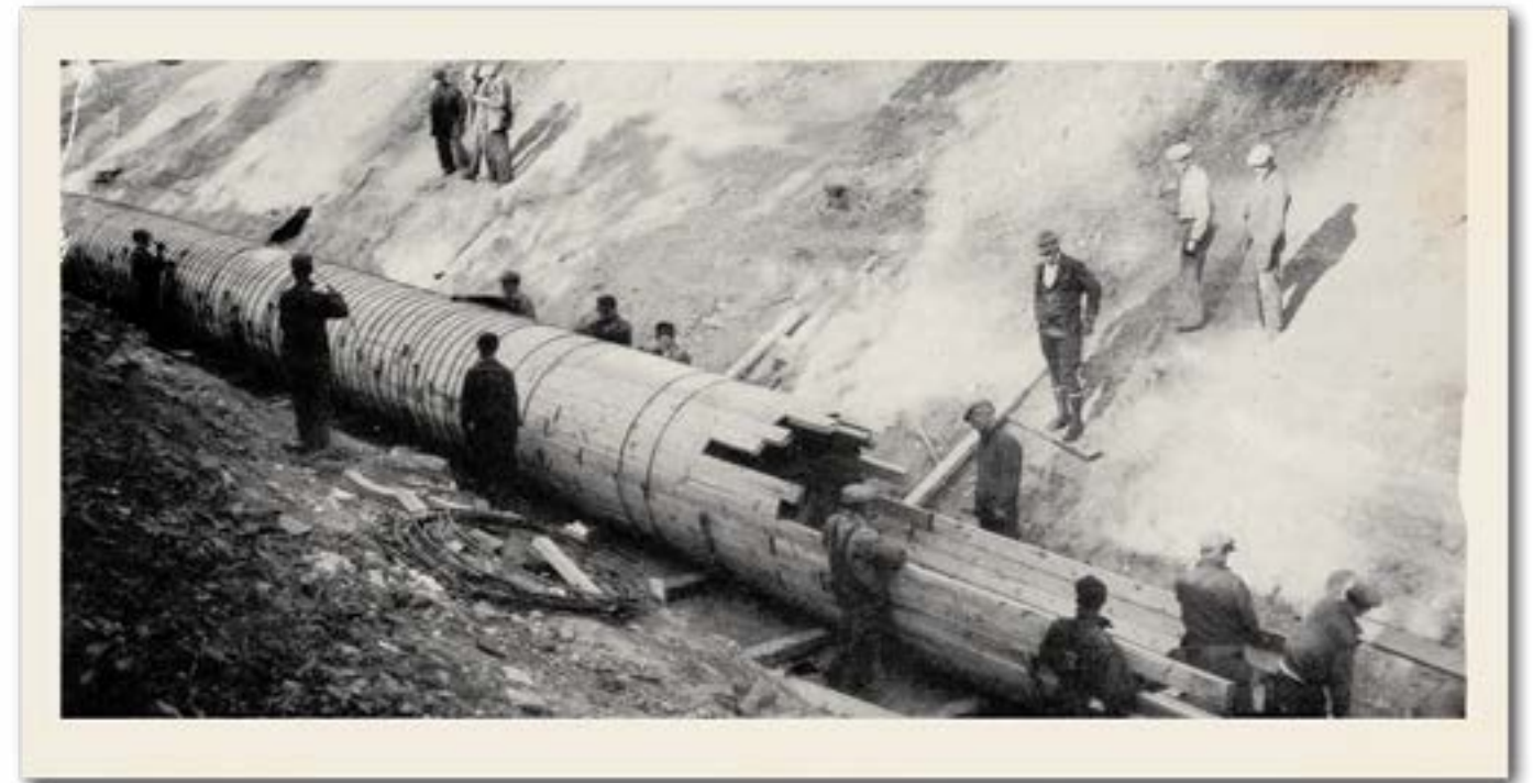
The wooden flume that carried water to the Big Bend Power Plant followed a five-mile route along Rapid Creek. It was built by hand using hundreds of laborers.
