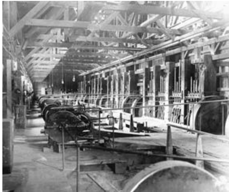
Equipment on the cam floor of the Gold Star Mill operated by the Homestake Mining Company. The first dynamo on Homestake property was installed in this mill in 1888 to power 75 lights.
