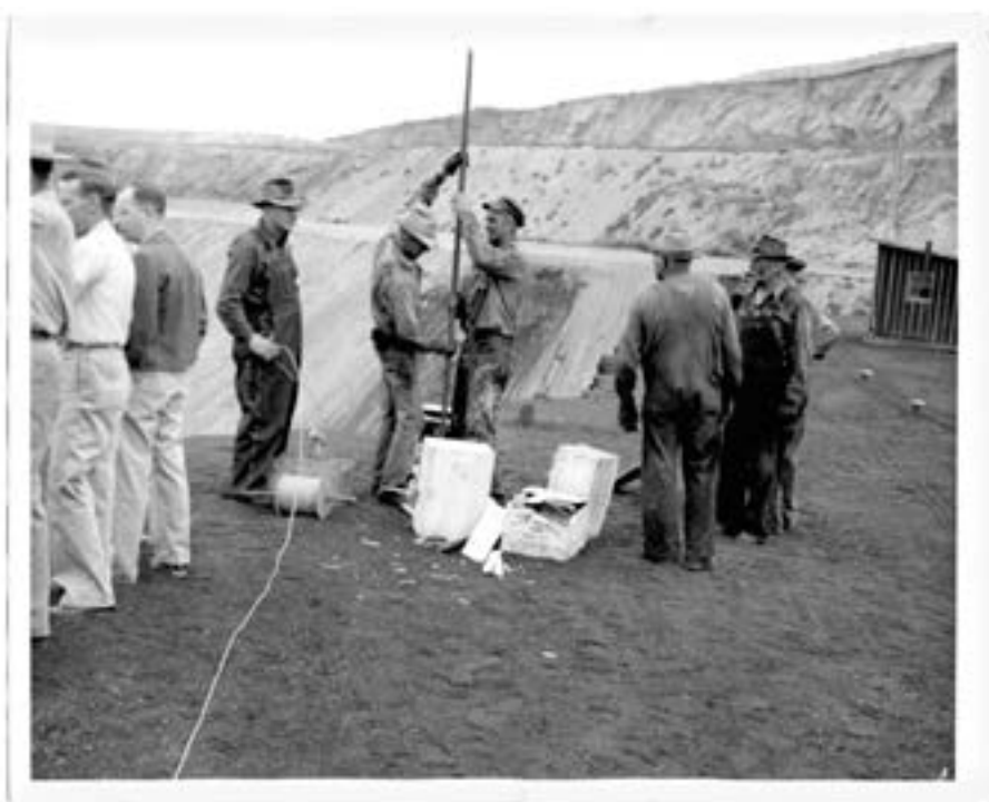
Wyodak miners charged a blast hole to loosen the coal for excavating. Using an auger, the miners would drill as much as 80 feet into the coal seam.
